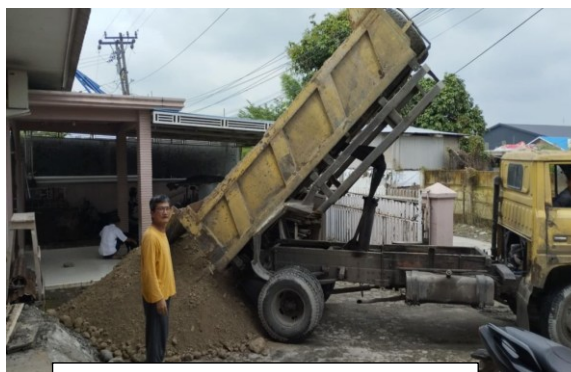
Unloading material for raising floor
