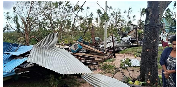
Destruction from Cyclone Yasa
